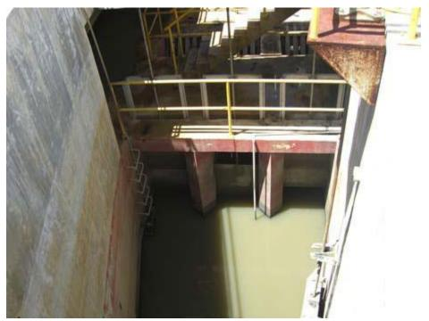
**History:** This activated sludge waste water treatment plant developed an historical serious problem from hydrogen sulfide, H2S, and experienced significant odor and corrosion problems. This plant processes 15 million gallons of water per day.
